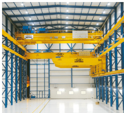
Double girder crane and cantilever crane
