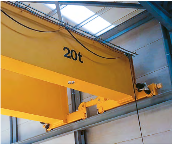
CRANE WITH DOUBLE END TRUCKS (EIGHT WHEELS)
